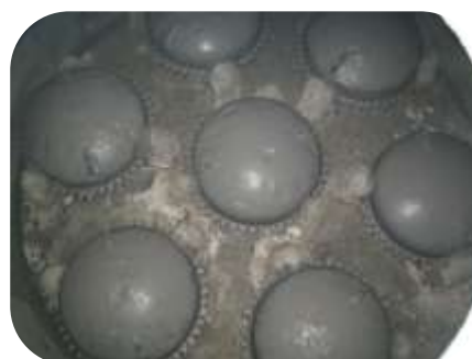
Ammonia distiller operating at 95-100°C had become badly corroded due to the harsh operating environment. The internal surfaces were abrasive blast cleaned and coat using 205 Ceramic HT Fluid
