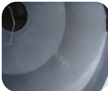
Process vessel operating at 95°C relined using 2 coats of 205 Ceramic HT Fluid
