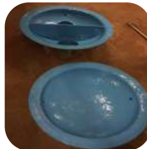
Heat Exchanger tube sheet, end covers and water box were all abrasive blast cleaned in situ to SA2.5 surface cleanliness. 201 Ceramic Repair Paste was used to rebuild any badly corroded areas and then all surfaces were coated with 2 x coats of 203 Super Flow at 300 microns per coat.
