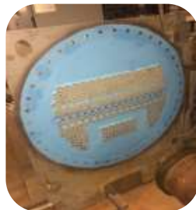
Heat Exchanger tube sheet, end covers and water box were all abrasive blast cleaned in situ to SA2.5 surface cleanliness. 201 Ceramic Repair Paste was used to rebuild any badly corroded areas and then all surfaces were coated with 2 x coats of 203 Super Flow at 300 microns per coat.
