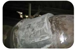
A hot chemical process line operating at 50° C was leaking around the flange fitting. He onsite contractor mechanically abraded the leaking pipe surface and cold bonded a steel plate to the repair surface. The steel plate was then over wrapped using 301 Epoxy Resin and Hardener and Glass Tape
