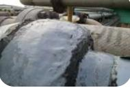
A live leak on a caustic line at a chemical plant required sealing. Previous repairs had failed. The flange fitting was abraded using mechanical grinders and encapsulated using 106 Metal Repair Paste XF
