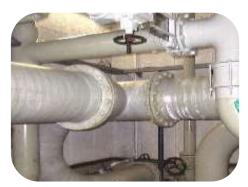
301 Epoxy Resin Hardener was brush applied to pipework situated in a plant room. The pipe wall thickness had deteriorated over time and the pipes were weeping hot water onto the floor below, Due to the fragile state of the pipes surface preparation was carried out using hand held wire brushes. Once the surface of the pipe had dried 301 Epoxy Resin and Hardener was applied at 1mm wet film thickness to the pipe surface and wrapped 3 times using 100mm glass tape
