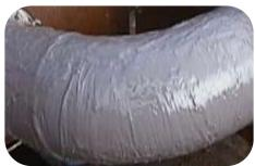
Diesel lines situated on a jetty at a refinery were leaking at the pipe socket. Using handheld scrapers and copper brushes the pipe surface was abraded by hand then coated using 104 Metal Repair Fluid XF
