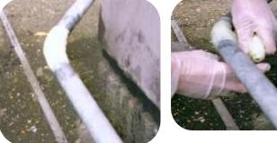
A chemical process line had started to leak due to a hole forming in the pipe wall, the surface was mechanically abraded and 108 Pipe Repair Tape wrapped around the pipe work to a minimum thickness of 12mm over the repair area.
