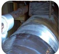
When used with 301 Epoxy Resin and Hardener 701/703 Glass Tape can be used to encapsulate isolated leaks or to encapsulate long lengths of large diameter pipe work.
