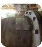
Leaking ammonia chemical line required sealing in an emergency. The surface of the pipe was mechanically abraded and a pre-formed steel plate bonded over the hole using 106 Metal Repair Paste XF. The repair was then overwrapped using 301 Epoxy Resin Hardener and Glass Tape
