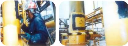
The bottom segment of a chemical process pipe had become badly corroded. The surface of the pipe was mechanically abraded using coarse grinding pads and a pre-formed steel plate cold bonded to the surface.
