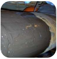
Ballast pipe on a 300mtr grain carrier had become so badly corroded the vessel was struggling to take on board ballast. Due to the confined space and restricted access the surfaces of the pipe could only be manually abraded. Once cleaned 302 Epoxy Repair Cement was applied to the repair surface. 301 Epoxy Resin and Hardener and Glass tape were applied once the repair paste had cured
